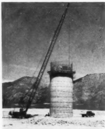
MODOC exhaust ventilation shaft rises above Berkeley pit waste dump.
